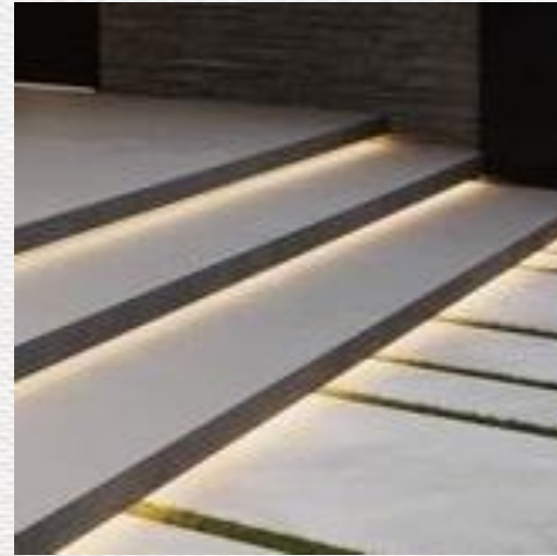
Stairs with LED lighting
